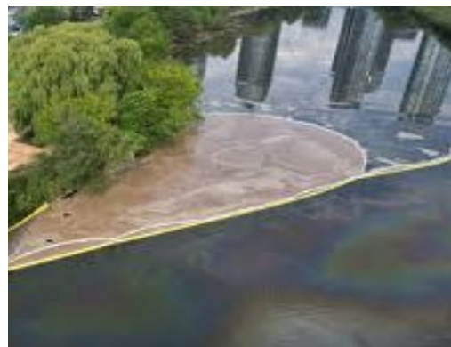
Photo2. Froth collector installed at the site in Mimico Creek
