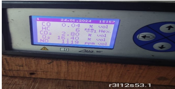
Fig. 7.2.3 Emissions diesel with hydrogen at 4ms
