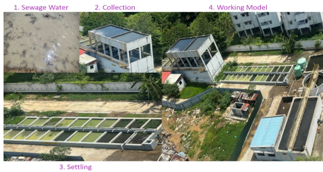
Figure 4. Real-Time Working Model Field Setup for Wastewater Recycling
