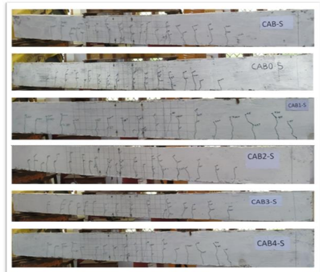
Figure 5. Crack Pattern and Failure Mode
