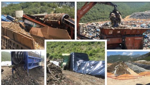
Figure 2. Mobile MBT facility in Kalamata, Greece.
