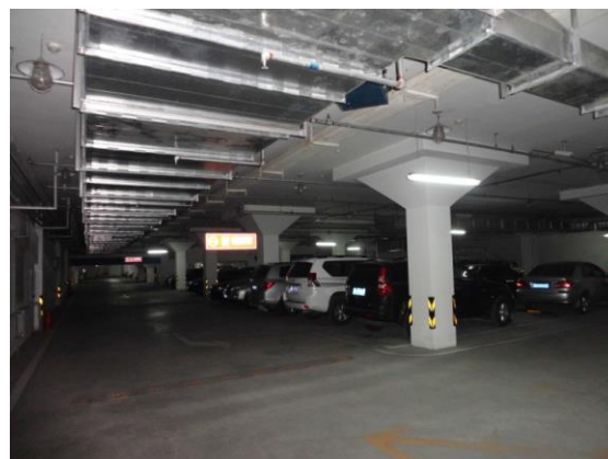
c) Environment inside the garage
