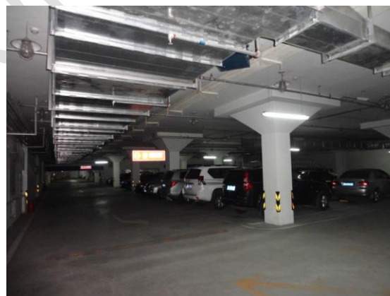
c) Environment inside the garage
