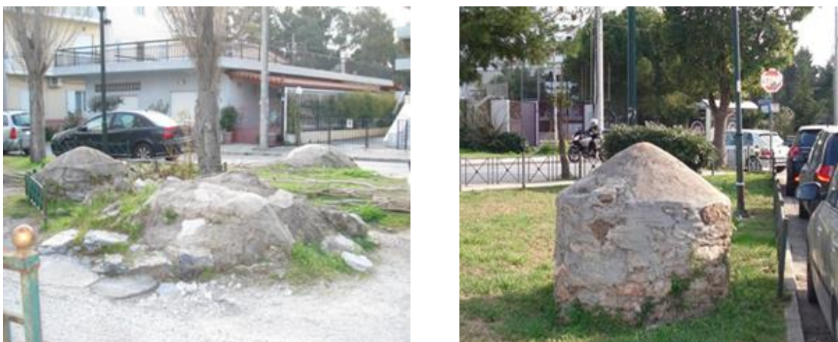
Figure 10. The beginning of Halandri transverse aqueduct. Wells at El-Alamein street, Halandri.
