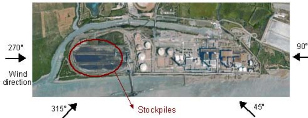
Figure 1. Top view of the industrial site
