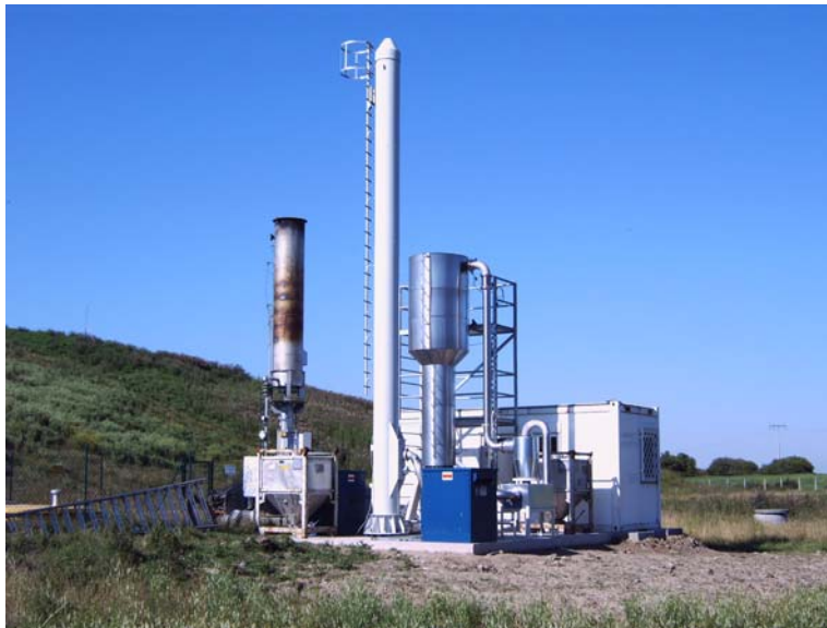
Figure 6. Construction of the SFBC on the landfill at Mecklenburg-Western Pomerania
